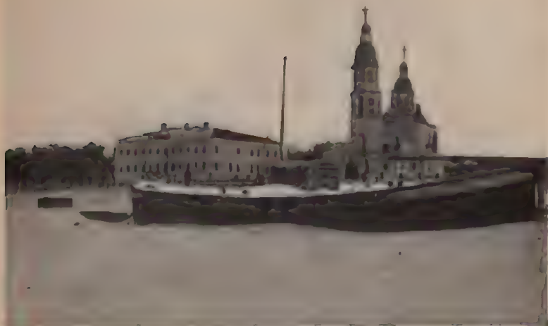
Looking across the frozen Dvina River to the American Red Cross Hospital (left) at Archangel, Russia.
